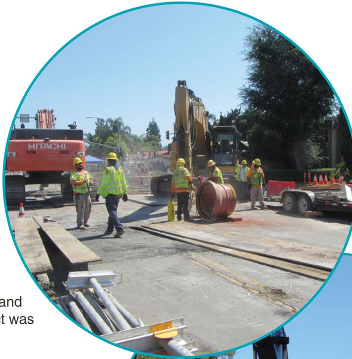
*(Left) 30-inch diameter pipe was installed along Red Hill Avenue, the Vitrified Clay Pipe was installed in segments each weighing approximately 2400 lbs. Pictured is the last piece of pipe installed which was smaller than the typical pipe segments used.*
