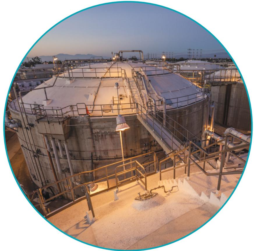
*The digesters at Plant No. 1 are approximately 30 feet high, have a diameter of 110 feet, and a capacity of 2.2 million gallons.*
